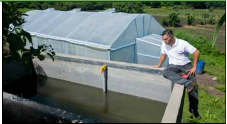
CRS agricultural technician Reynaldo Centeno checks the water level of a storage tank in the Sébaco area of Matagalpa Department. The tank uses a gravity-fed system to water seedlings in the ACORDAR greenhouse as well as the farmer's crops beyond. Rick d'Elia for CRS
